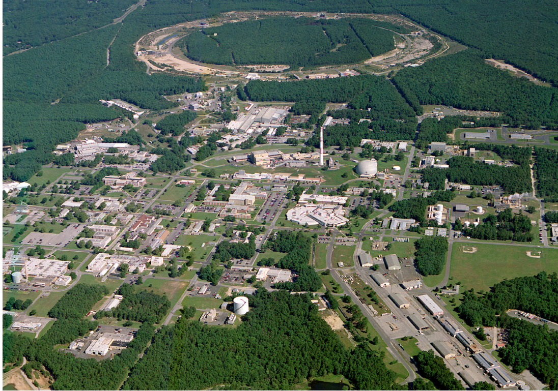
Figure 4.1: This is an ariel view of the RHIC facility in Upton, NY, facing north. Note the RHIC ring is in the background. The facilities directly producing or accelerating the colliding beams are in the top half of the picture, with the first such facility in the chain being the Tandem van de Graaff building just above the middle.
